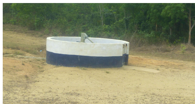
Figure 2: Non-functional School hand pump requiring only a U-seal replacement (Grand Cape Mount, March 6, 2019).
