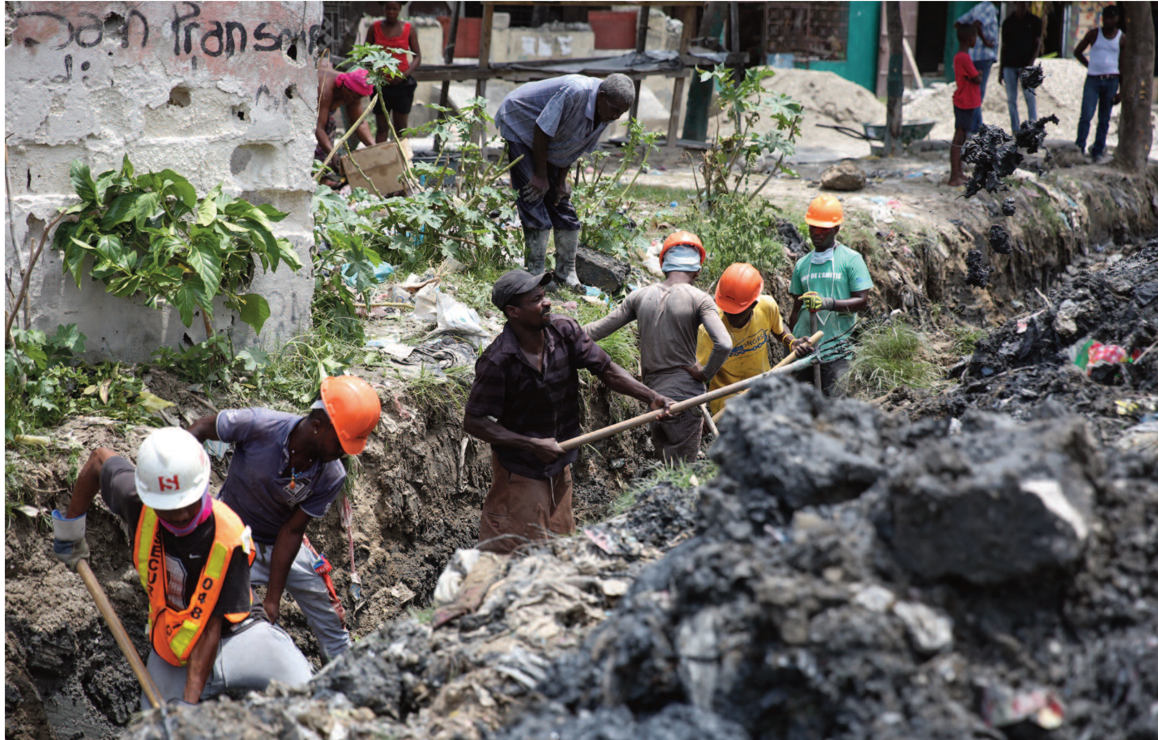
Drainage canal clearance work in Port-au-Prince, Haiti. Rubbish washed down from the city blocked these canals causing flooding and disease in low-lying communities.
