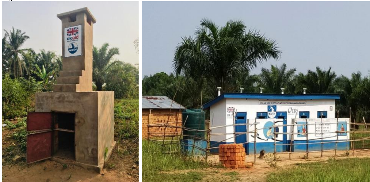
Figure 2: DRC WASH Consortium–Facilitated Sanitation Infrastructure in Kasai Central
