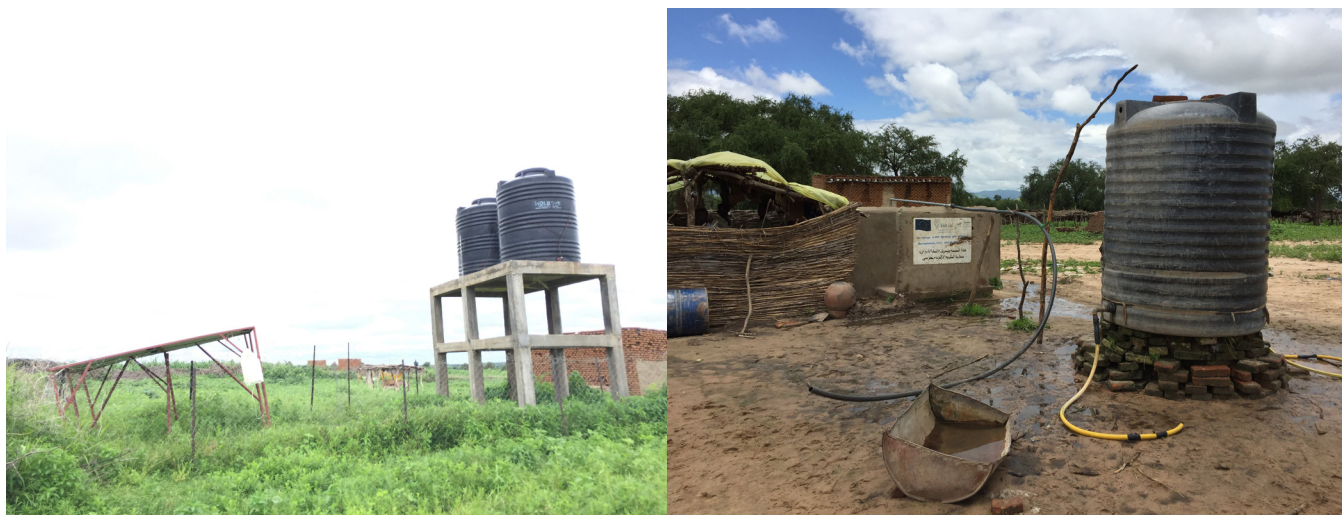
Photo 6: Solar-powered borehole in Maramara (left) and motorized pump borehole in Tcharo (right)
