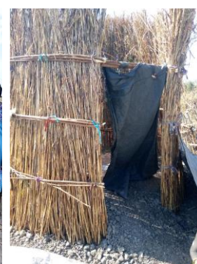
Figure 5: A completed latrine constructed by community members with local materials.
