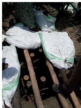
Figure 1: A completed pit under lining in Kurkal
