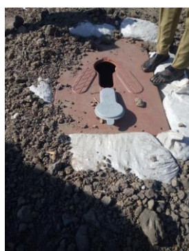
Figure 3: A lined pit with slab.
