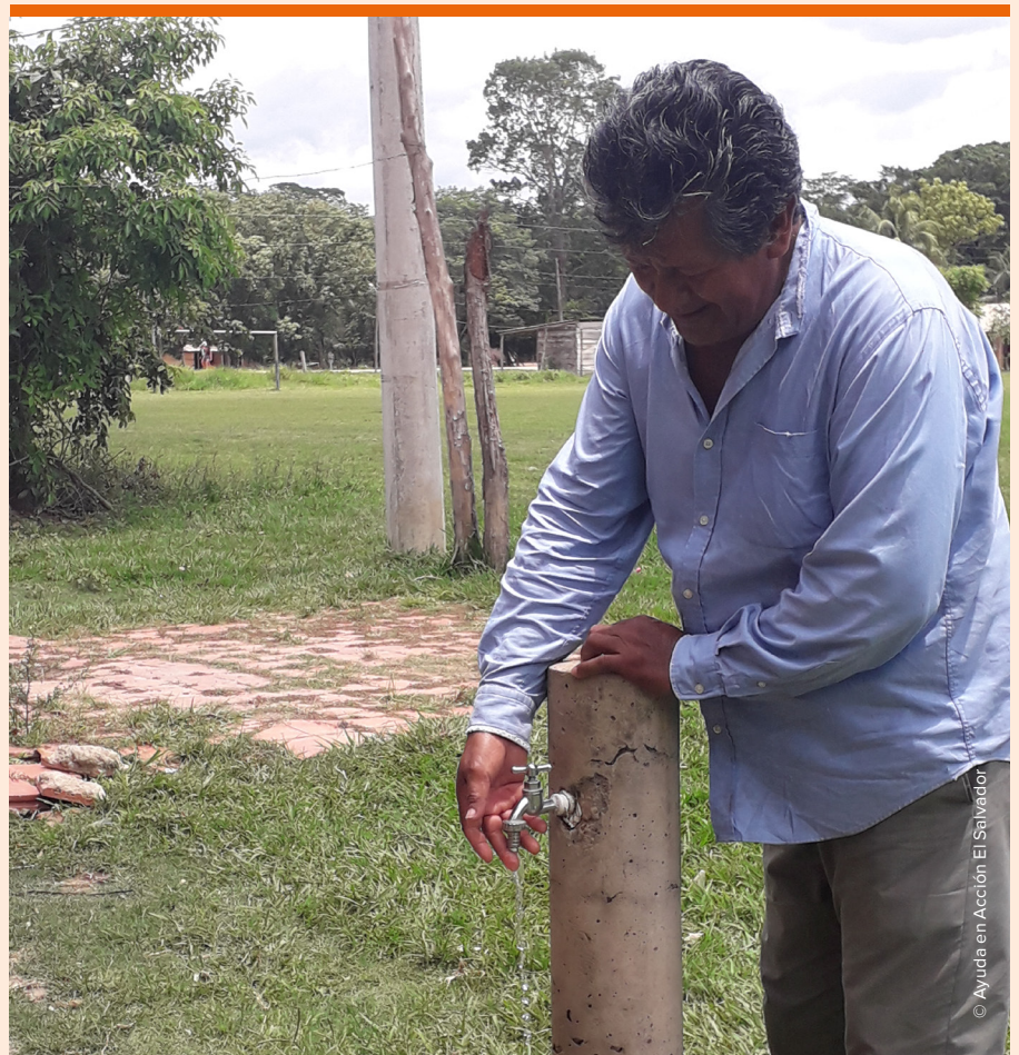
Bolivia, Photovoltaic system for water distribution in the Tarija Chaco region.
