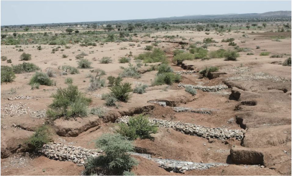
Figure 3: Gabion check dam showing partly replenished soil levels near Satille village, Borama, Somaliland. Photo: Mohamed Ahmed Ibrahim/Concern Worldwide.
