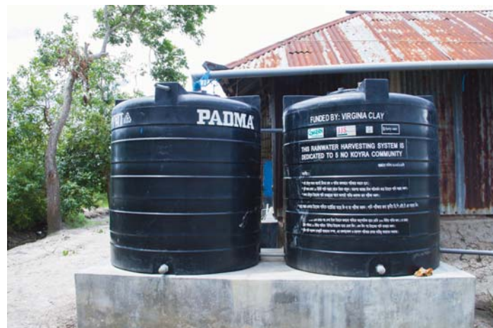
A community based Rainwater Harvesting System with a storage capacity of 4000 litres in Shymanagar, Satkhira
