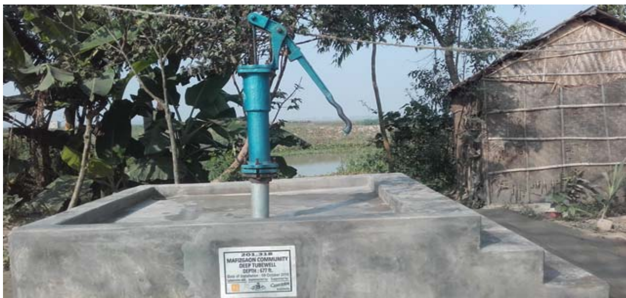
A deep tube well with raised platform installed in Mithamoin, Kishoreganj, which serves almost 100 people in this community.
