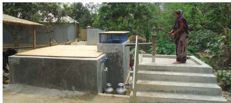
A woman using a community based Arsenic Iron Removal Plant in Bagha, Rajshahi.
