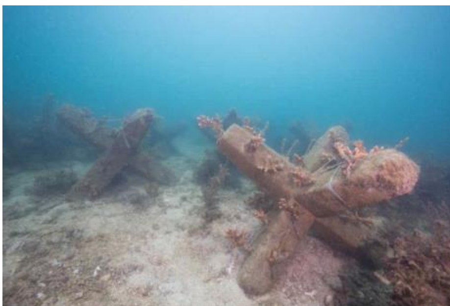
Figure 4: Concrete artificial reef with transplanted coral fragments
