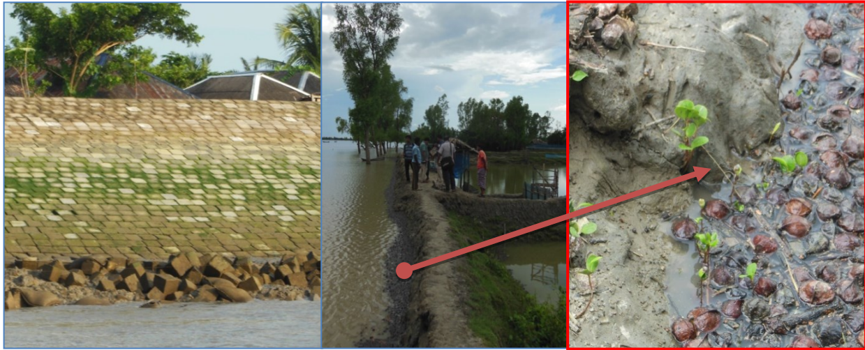
Residents of Bangladesh use a number of different types of embankments, including large and strong embankments (left) and smaller ones (centre and right). The larger embankments provide a greater level of protection but at a higher cost. The smaller ones offer protection from small scale hazards that occur frequently - the one pictured prevents agricultural land and settlements from becoming inundated monthly during high tide when the moon is full (spring tides) - but only offer marginal protection from larger hazards. Trees were not planted following the construction of this embankment, but mangroves are beginning to take root, their seeds being naturally swept to the embankment by the moving current.
