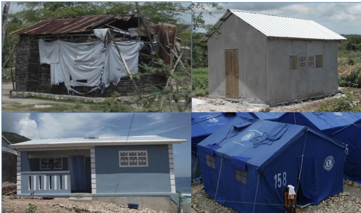
These pictures show a few different house styles used around La Gonâve. On the upper left is an example of a poorly constructed traditional house found on the island. The house offers little protection from the elements and would not last through a small storm. On the upper right is a temporary house built by Concern. It costs more than a tent (below right, photo credit the Lions Club) but is much more robust and maintains a better temperature. The house on the lower left is a permanent house built by Concern. Before Concern's involvement these houses were being built using salt water to mix concrete, increasing rates of rust of the reinforcement bars and reducing their lifespan.
