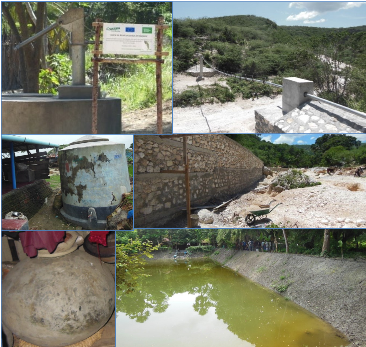
These pictures show some of the ways Concern improves water. In Mozambique (upper left), Concern rehabilitates and rebuilds water points that are damaged or in disrepair, constructing points on a raised platform to reduce exposure to floods. In Haiti (upper and middle right), Concern goes to great lengths to hazard proof its water points and deliver water to communities in need. These pictures show a water point being repaired. The point is located in a gully, so is being built to withstand floods, in addition to earthquakes and storms. In Bangladesh (middle left and below), Concern’s work focuses on improving surface water as groundwater is salinised and often contaminated with arsenic. In some cases, Concern will help improve ponds (right below), and in others it will help households shift from traditional collection and storage techniques (left below), to improved techniques (left middle).
