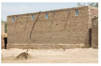
A reconstructed house in Pakistan: constructed on a plinth, the bottom third is waterproof, the top two thirds are mud brick. (Photo Dom Hunt 2012)
