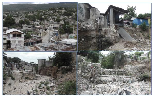
A number of houses near the gully in the Grand Ravine have been destroyed or are threatened by erosion. Concern constructed two check dams to reduce gully erosion, however they are showing signs of wear (bottom right photo).
