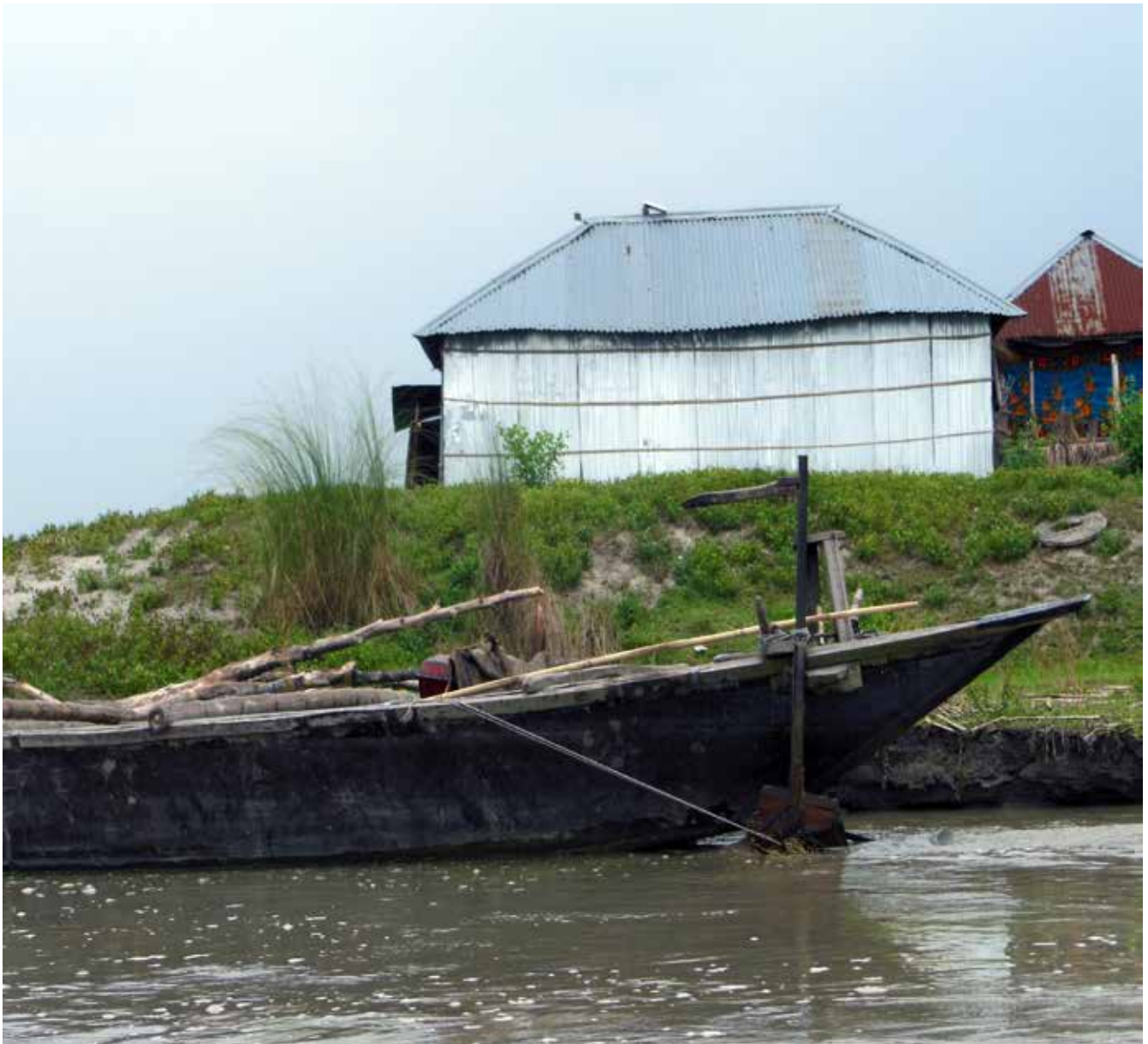
Settlement on a riverine island in northern Bangladesh. Houses are built on raised plinths to keep them dry during the months of high water. Concern also assists people to to develop vegetable gardens and plant fruit trees on the plinths, as well as installing latrines and wells. Photo by Aaron Clark-Ginsberg, 2013
