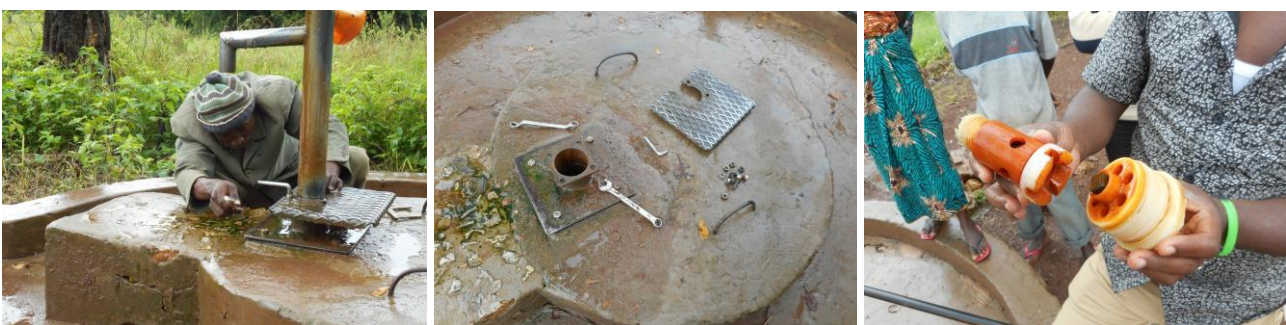
Figure 15. Pump caretaker for PE17 dismantling pump showing the Nira AF-85 foot valve.
