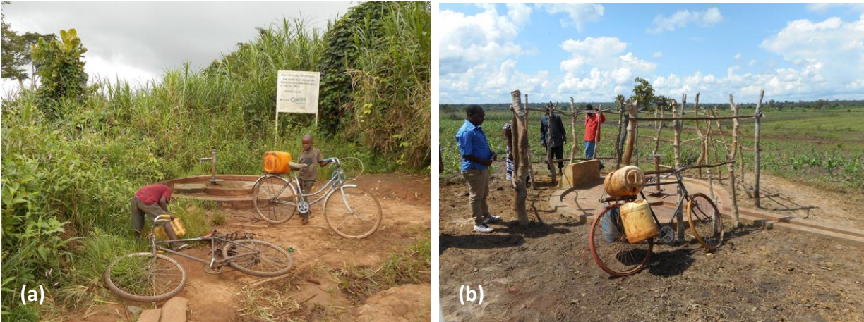
Figure 12. A tale of two water points: (a) PE15 – 6 years of operation without maintenance (b) PE11 – dry for most of its 14 months since installation and not used by community.
