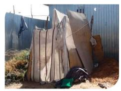
Figure 5: Collapsed Latrine
