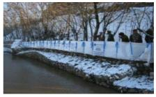
Above: Flood defence made from geotextile cells filled with earth. Photo by Tom Dobbin 2012.
