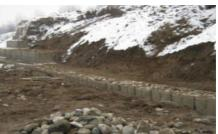
Above: Landslide-prone slope stabilised using Hesco cells. Photo by Tom Dobbin 2012.
